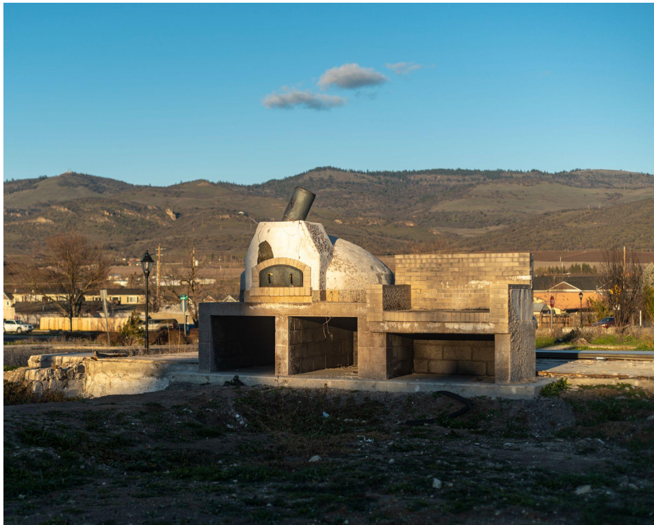
[Eden McCall, A chimney is all that's left of a commercial building in downtown Talent, Oregon, February 2, 2022]
