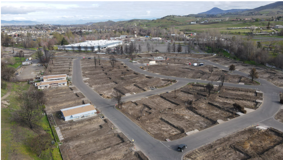
[DOT, "Drone view of Mountain View Estates Mobile Home Park in Talent, Oregon," April 8, 2021]
