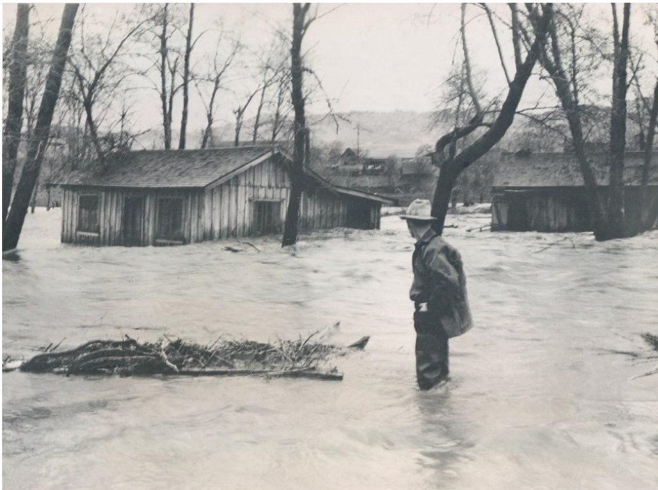
[Southern Oregon History, "Bear Creek floods the Talent area, February 28, 1940]
